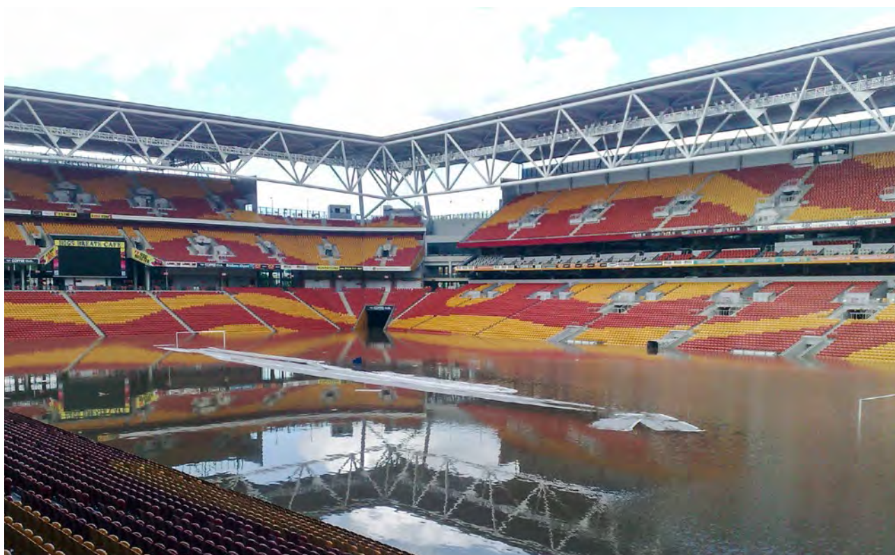
Figure 13: Lang Park (Suncorp Stadium) in Brisbane submerged after intense rainfall and floods in January 2011.
